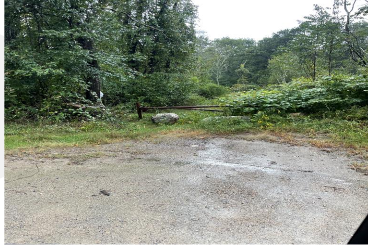
Inadequate Trail Widths
